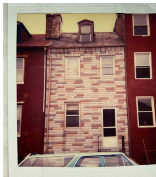
Begin with Formstone, end with brick.
