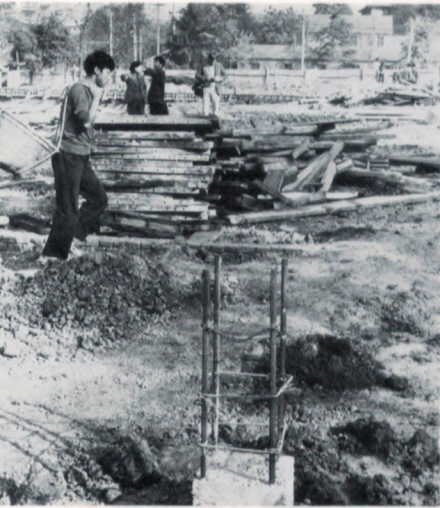
Construction workers haul dirt out of the foundation site.
